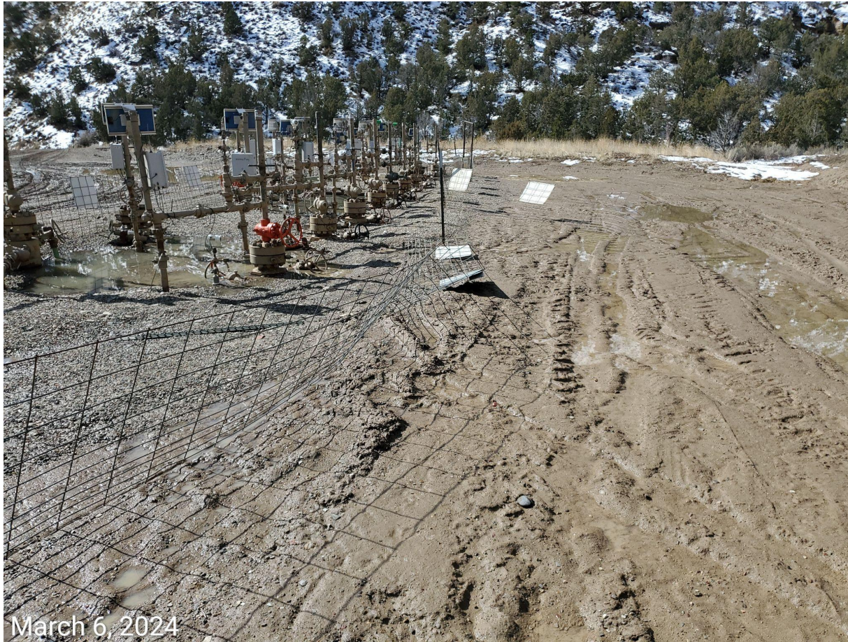
Photo 7: Fencing at wells in disrepair.
