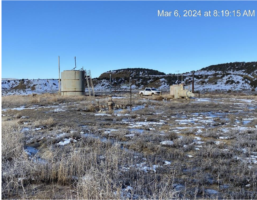
Location from Southeast corner
