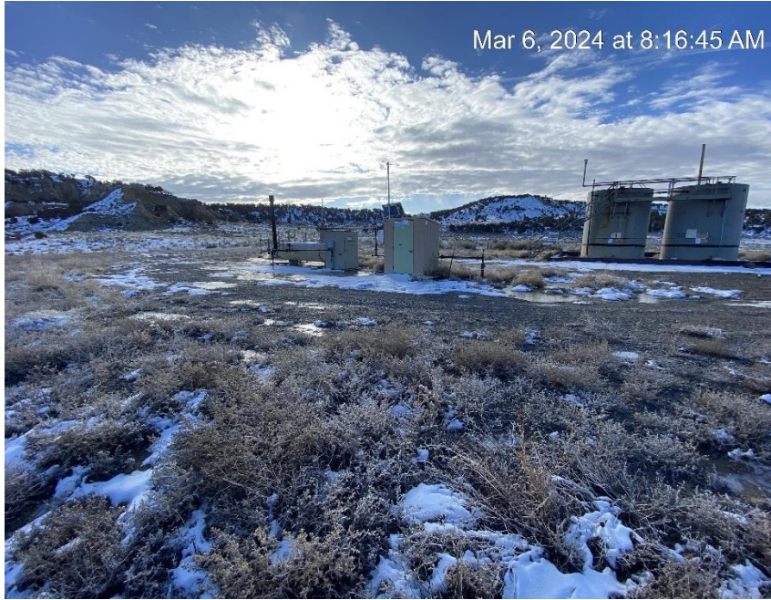
Location from Northwest corner
