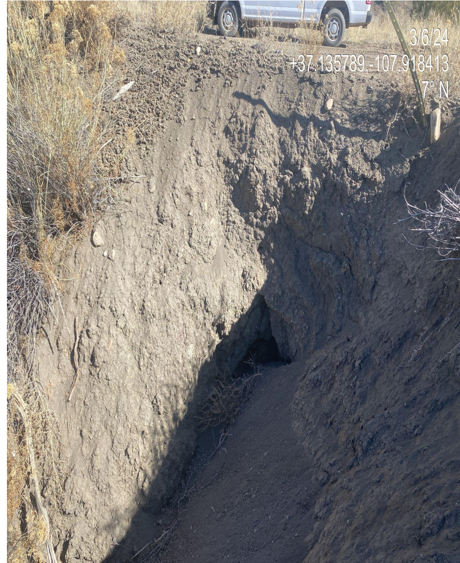
Photo 3. View of gully erosion forming on the western edge of the disturbance at the access point. Erosion is tunneling through exterior berm and causing additional erosion and sediment transport off of the location.
