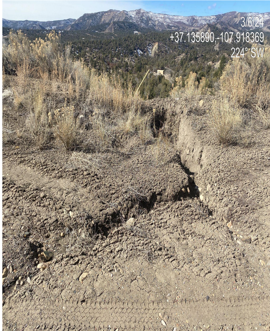
Photo 3. View of gully erosion forming on the western edge of the disturbance at the access point. Erosion is tunneling through exterior berm and causing additional erosion and sediment transport off of the location.
