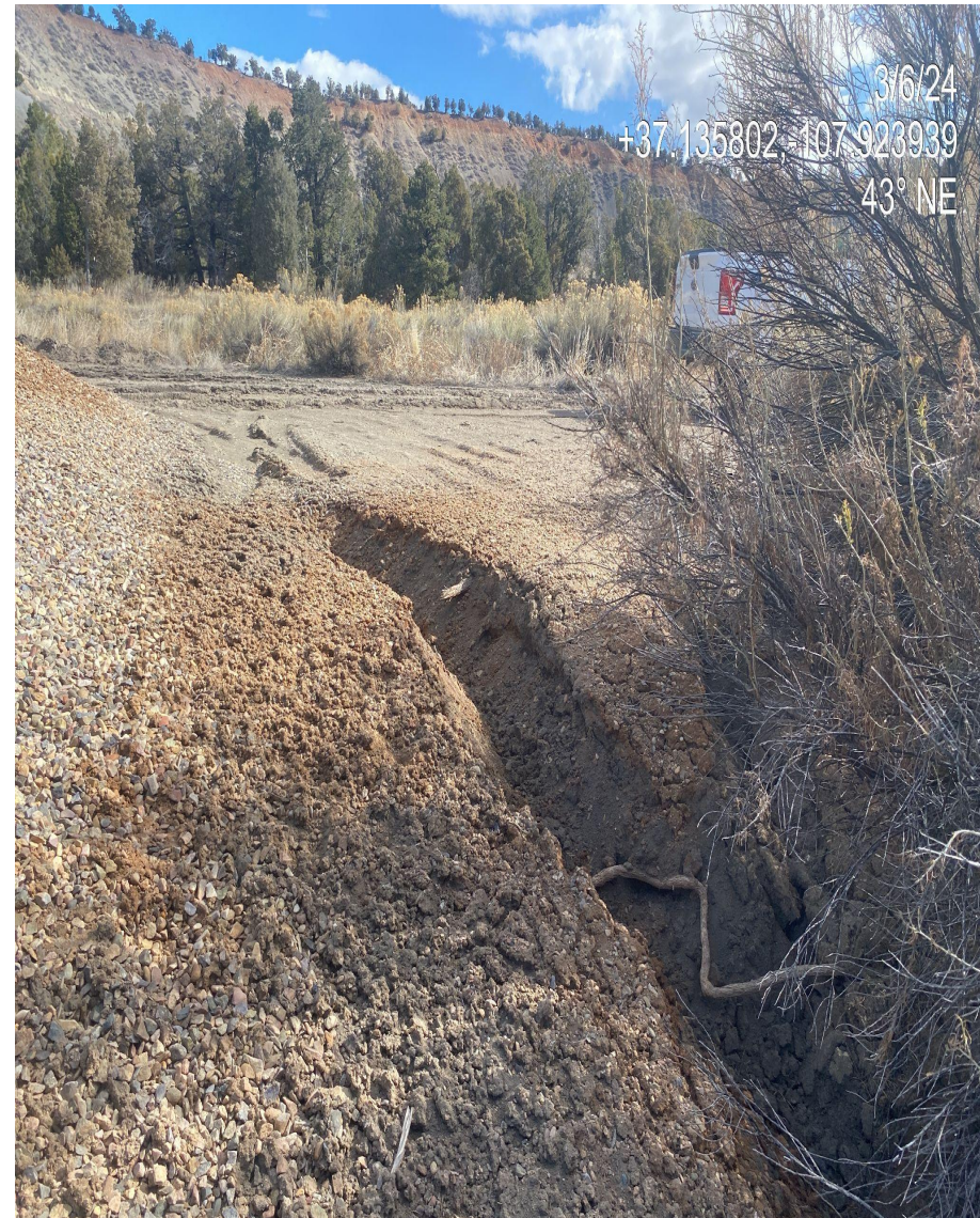
Photo 5. View of gully erosion forming on the western edge of the disturbance.
