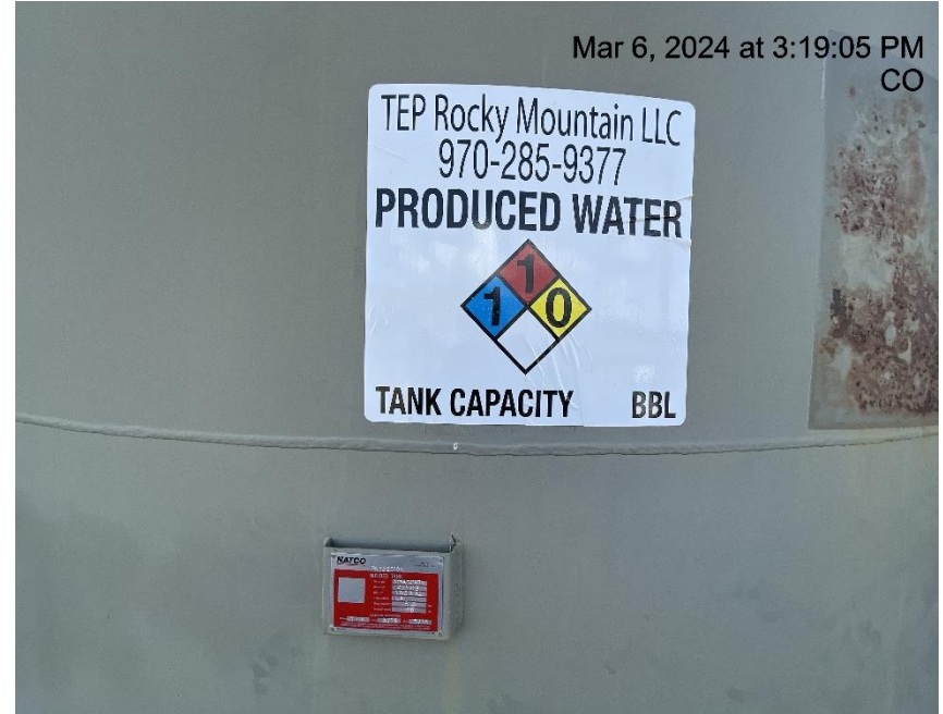
Photo # 8544 Tank label missing required information
