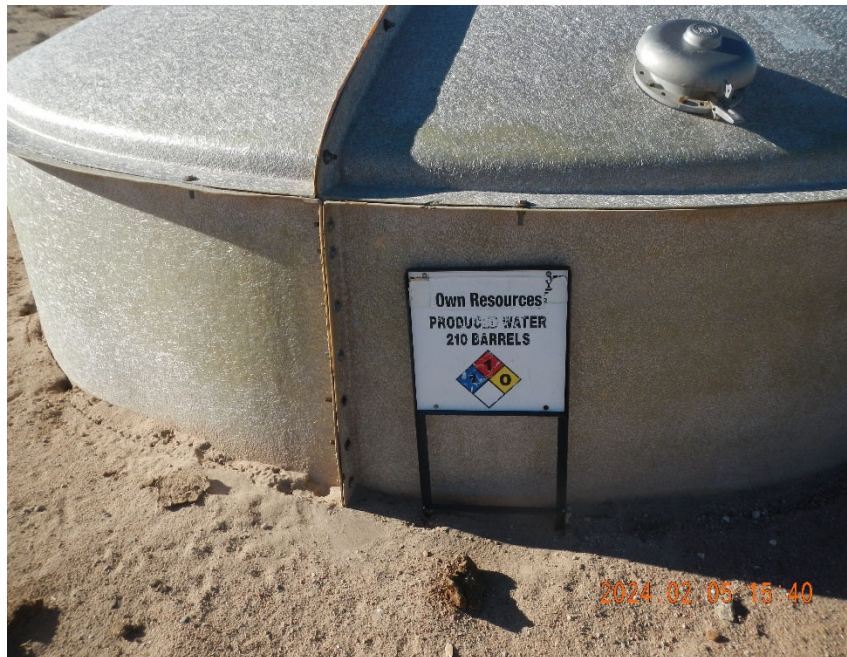
3. Produced water tank at well location.
