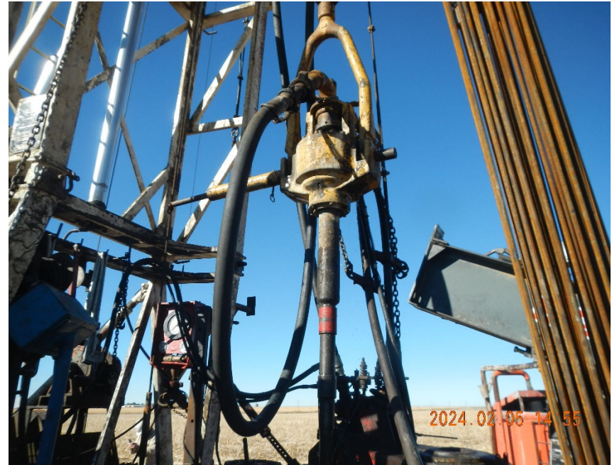
4. Power Swivel hanging from mast and drilling out CICR.
