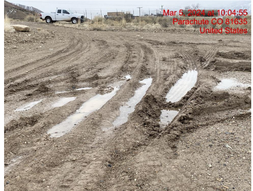
Lack of Stabilization/Insufficient Vehicle Tracking BMPs at Location Entrance/Exit – Photo #09695
