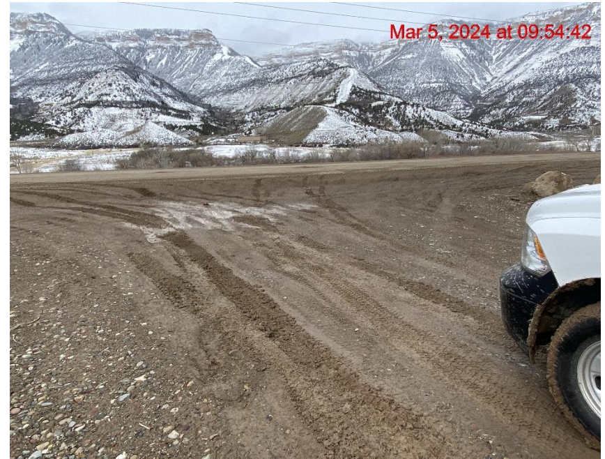
Insufficient Vehicle Tracking BMPs at Location Entrance/Exit – Photo #09689
