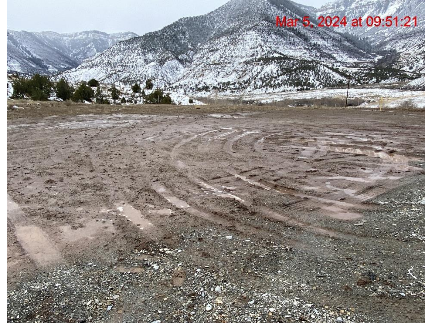
Lack of Stabilization – Photo #09683
