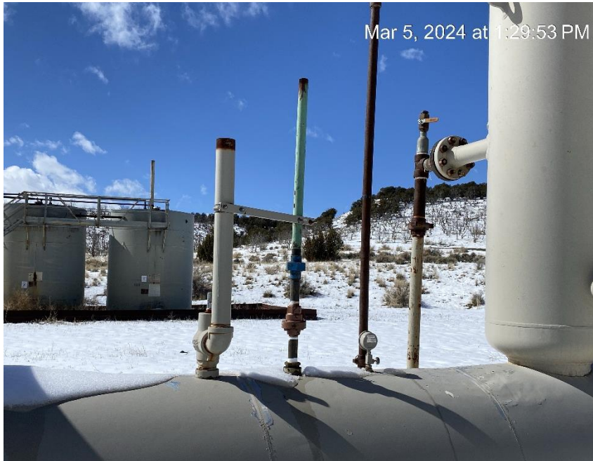
Relief missing rain cap
