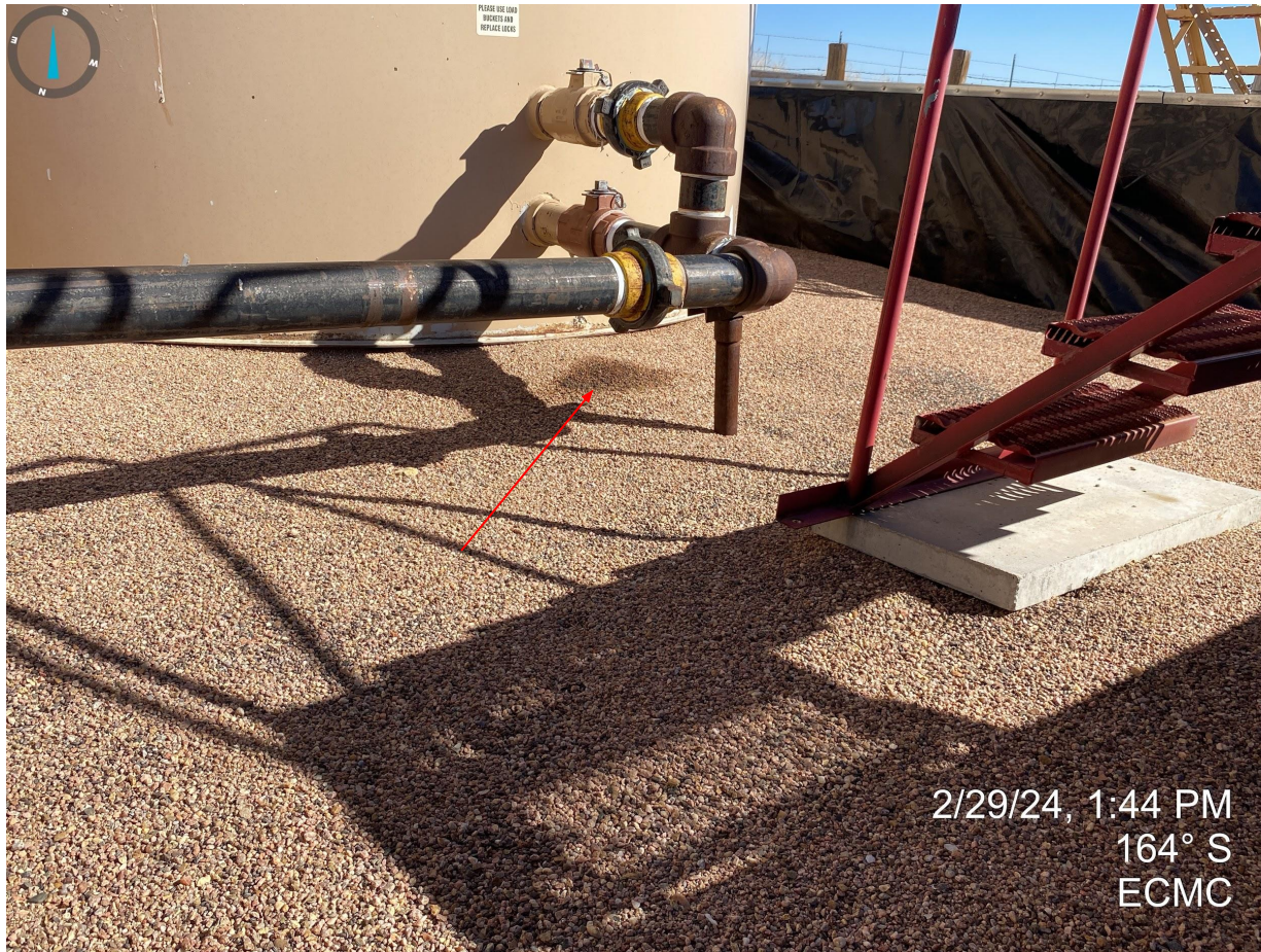
Photo 4. Stained soil observed at southern vertical steel tank.
