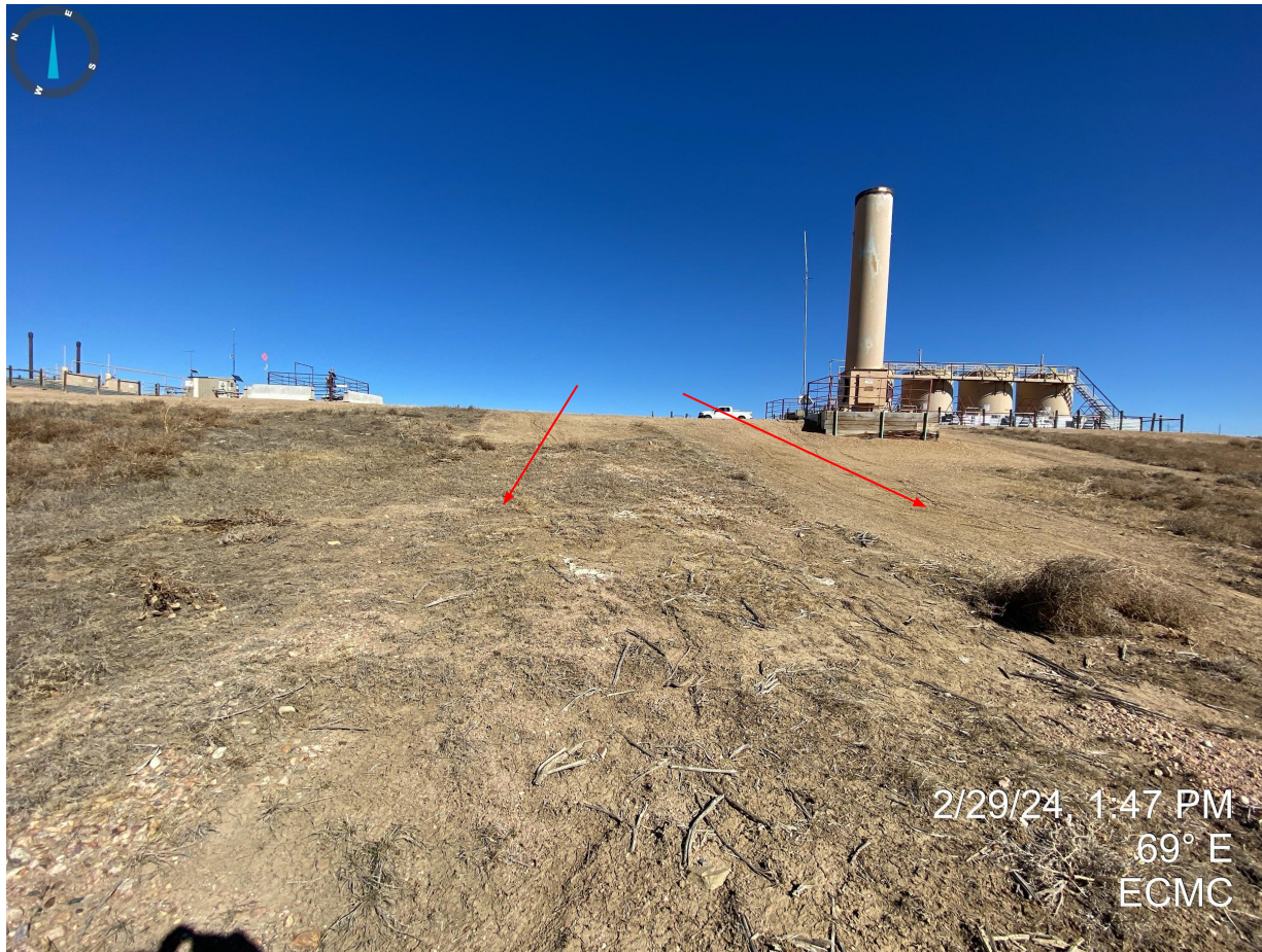
Photo 7. Western portion of location. Erosion degradation appears to have been repaired previously; no apparent stormwater control measures/BMPs observed to manage stormwater runoff. Bare soils require additional reclamation activities to stabilize the soils.
