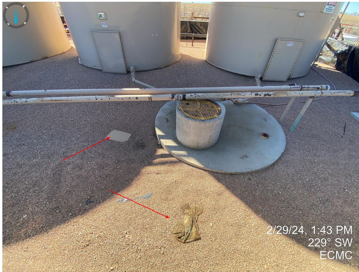
Photo 1. Debris within tank battery secondary containment.
