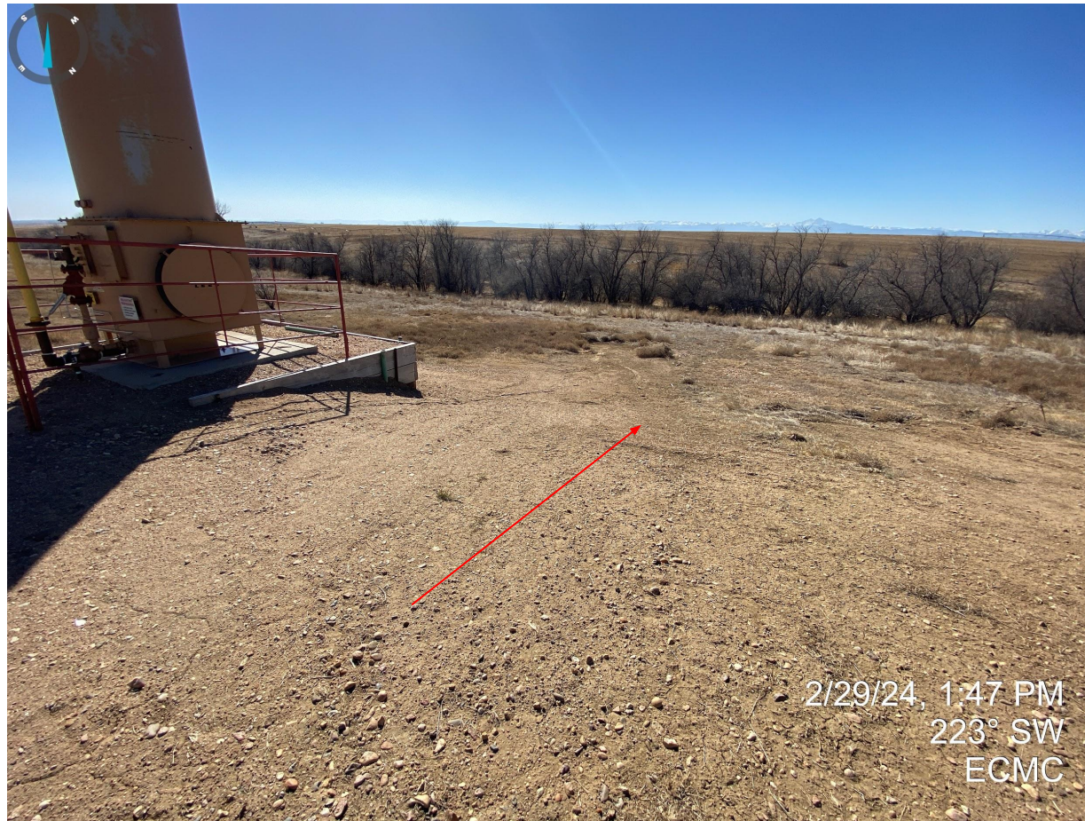
Photo 8. Western portion of location. Erosion degradation appears to have been repaired previously; no apparent stormwater control measures/BMPs observed to manage stormwater runoff. Bare soils require additional reclamation activities to stabilize the soils.
