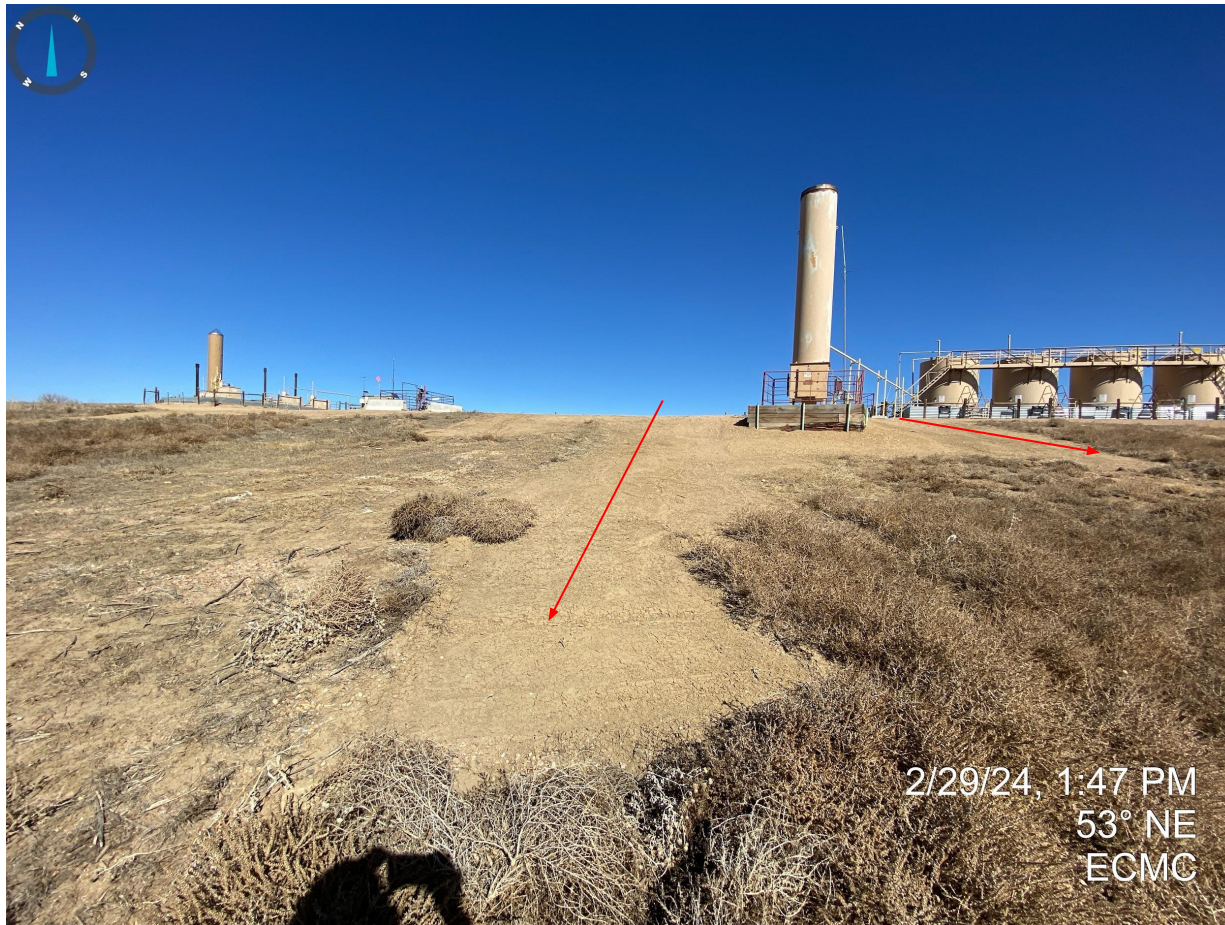
Photo 6. Western portion of location. Erosion degradation appears to have been repaired previously; no apparent stormwater control measures/BMPs observed to manage stormwater runoff. Bare soils require additional reclamation activities to stabilize the soils.
