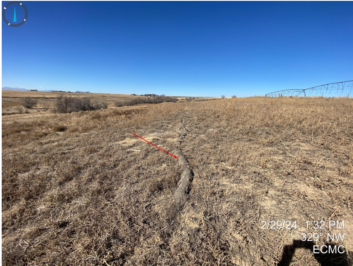
Photo 1. Debris (straw wattle) remains on location and will need to be removed.
