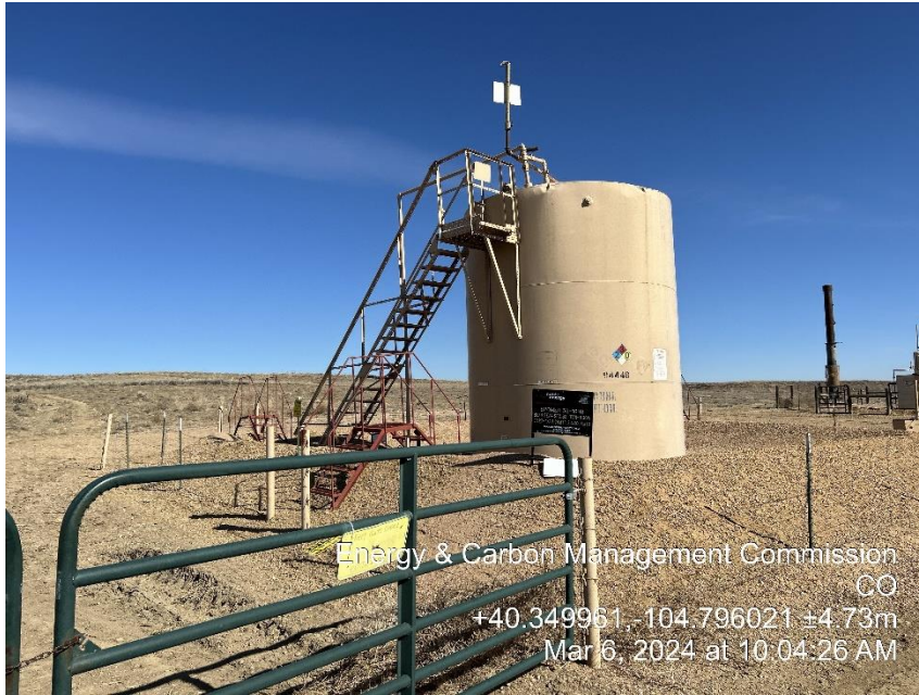
Photo 3 Tank battery
