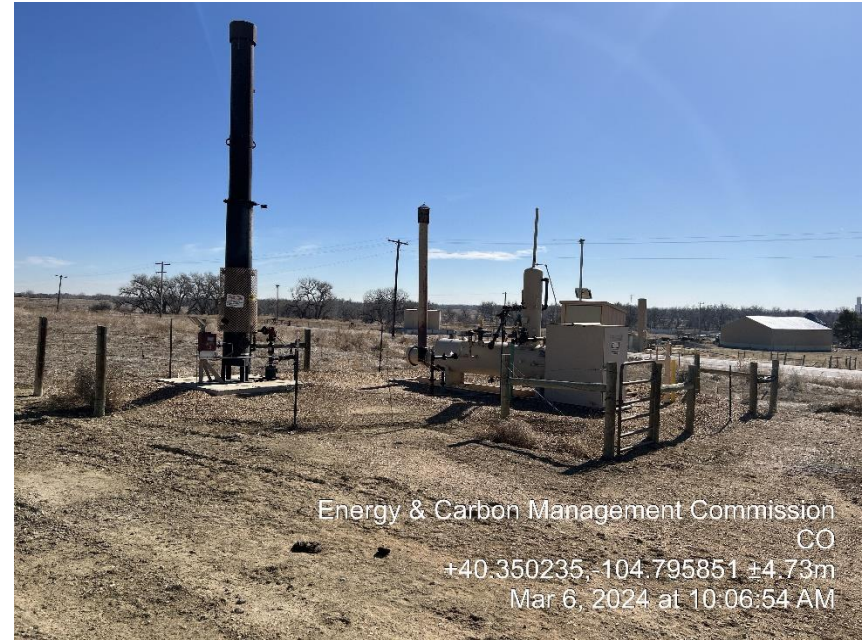
Photo 4 Separator/ECD
