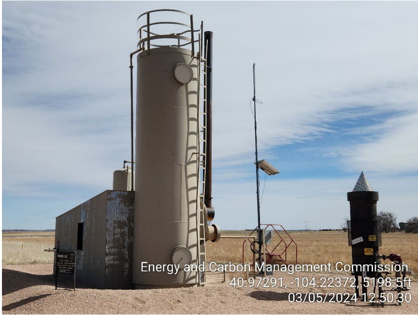
Photo 1 – Heater Treater and ECD
