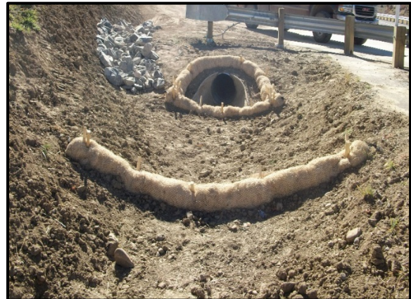
Erosion Logs along construction access road
