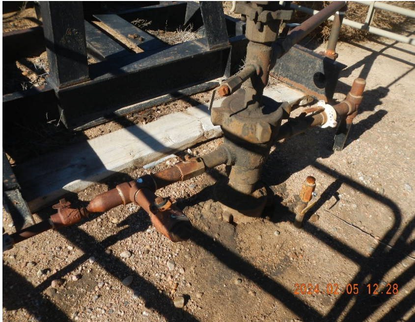
3. Additional view of wellhead. Note stained soil around wellhead.
