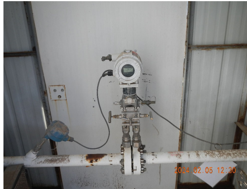
6. Digital gas meter inside meter shed.
