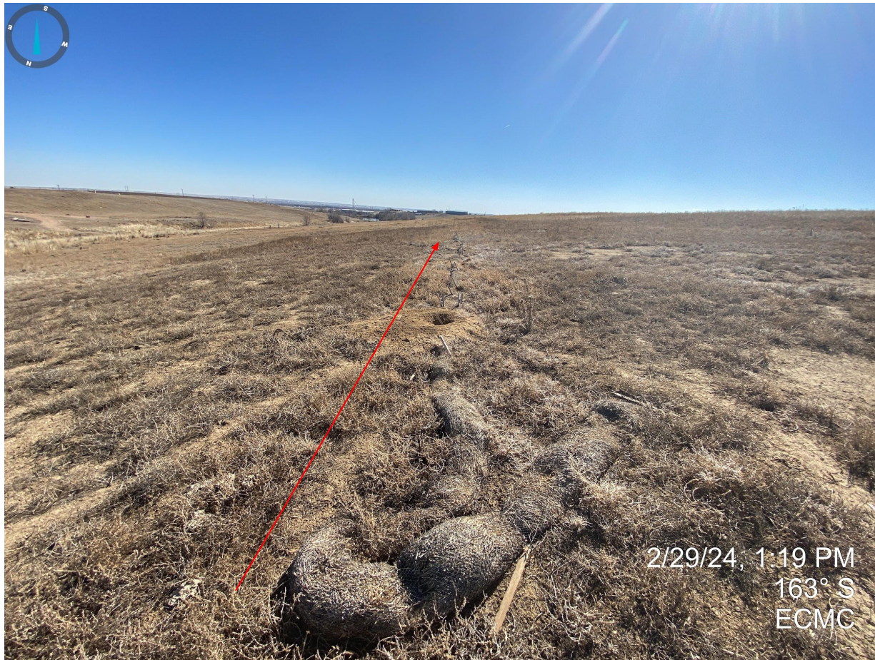
Photo 6. Degraded straw wattles and stake on location are now considered debris and require removal.
