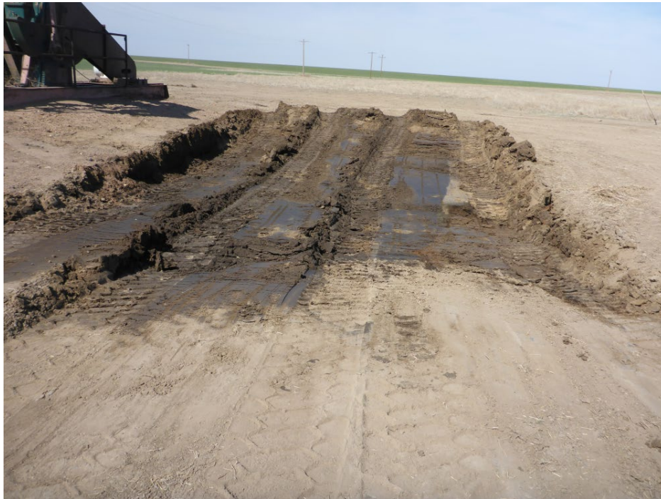
Begin excavation at Sample point V1A-N Venrick #1A (looking West)
