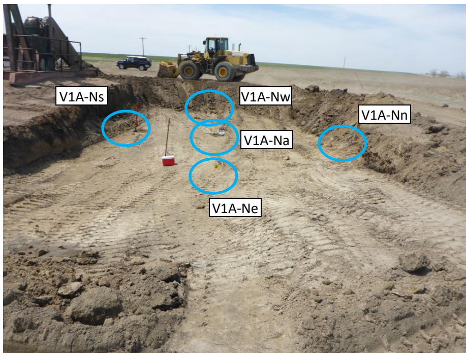
North side excavation – Sample points for closure Venrick #1A (looking West)
