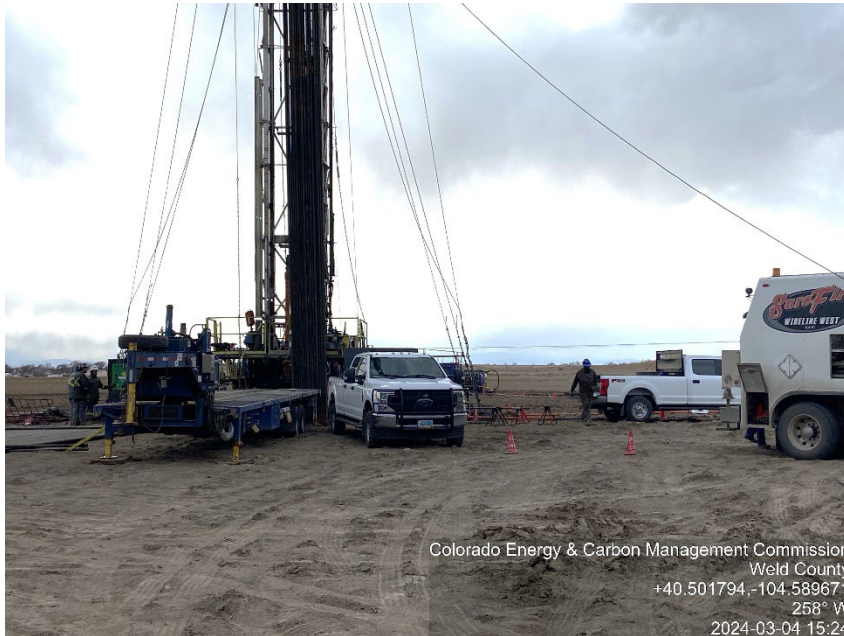
Photo #1 Ehrlich 32-7 (123-20196) Wellsite Plugged & Abandoned | PA Plugging Ops; Cementing: initial plugs
