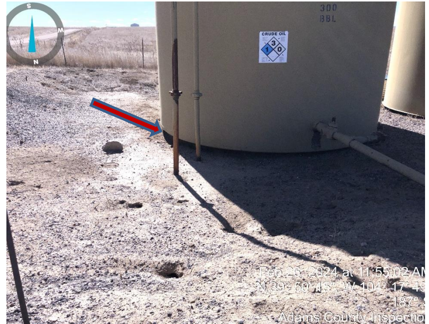
Photo #2 base of containment eroded under tanks.
