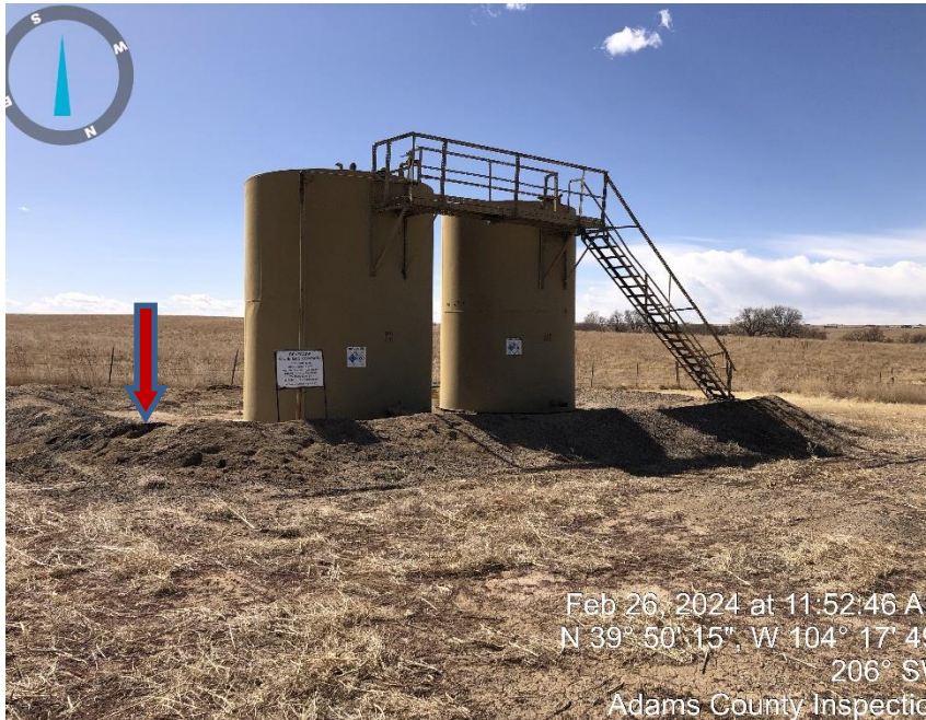
Photo #1 tanks and berm that needs maintained.
