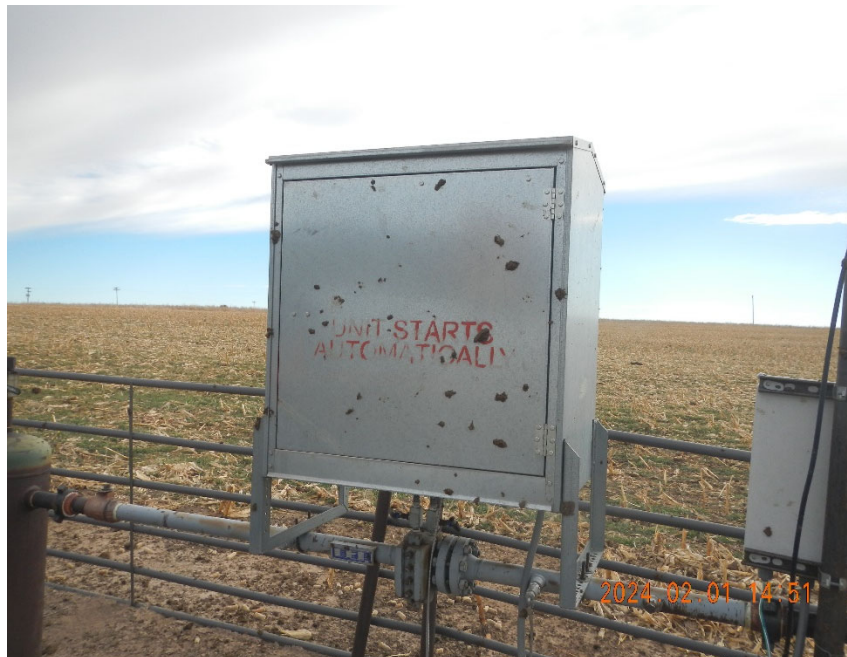
3. Flowline mounted gas meter run box.
