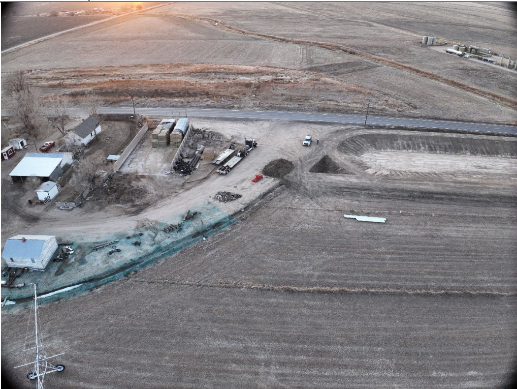
In View – Tank Battery, Flowline
