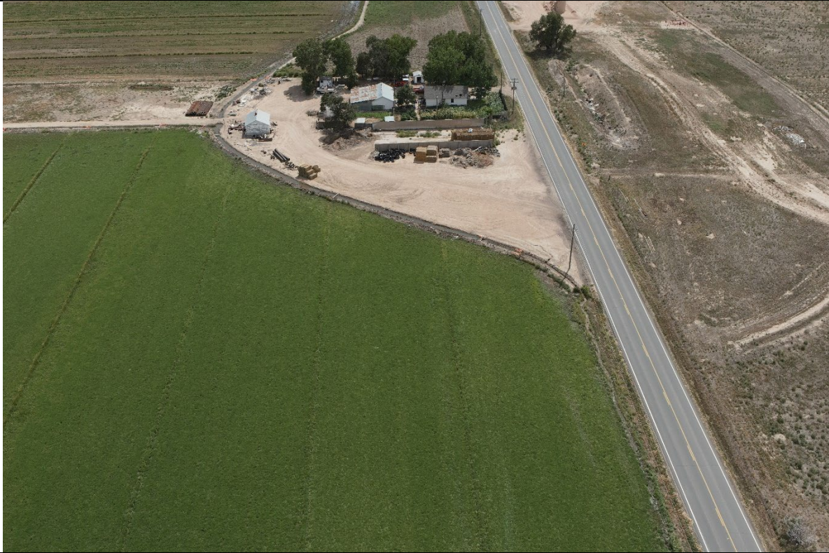
In View – Tank Battery, Flowline
