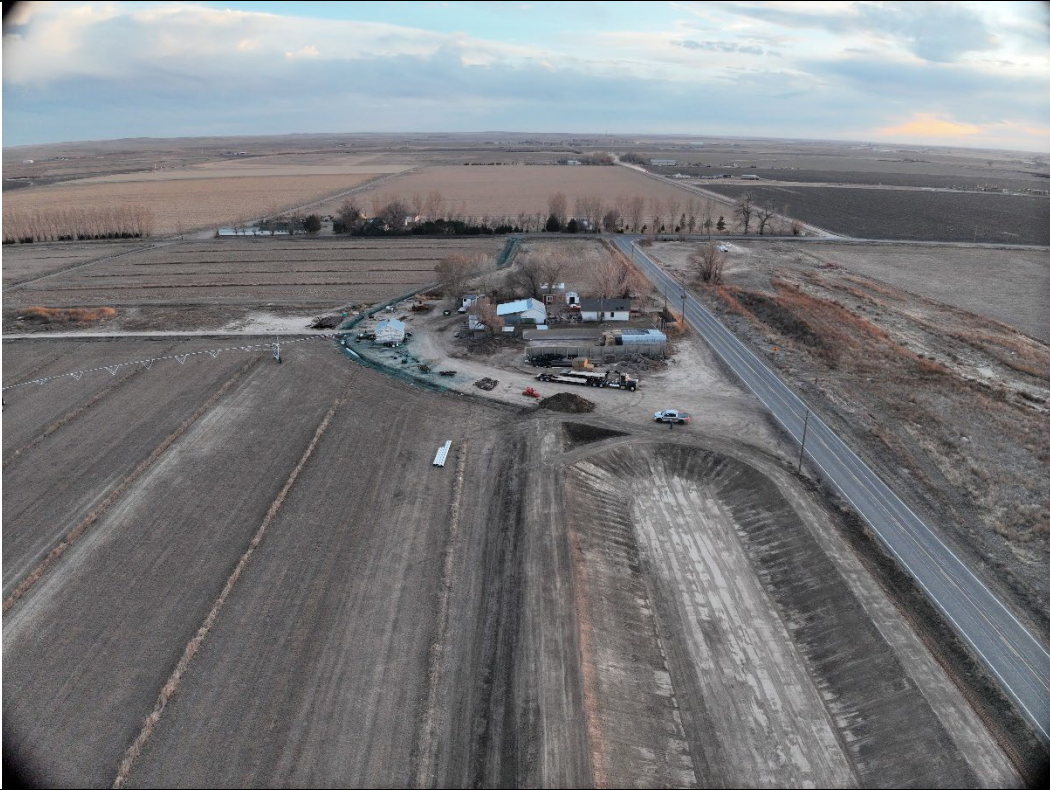
In View – Tank Battery, Flowline
