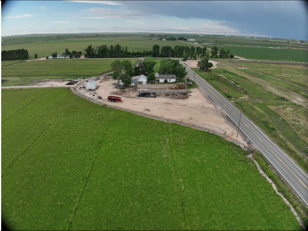
In View – Tank Battery, Flowline
