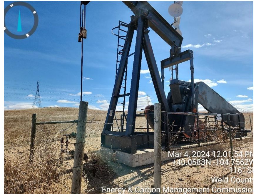
Photo 4 well head and equipment
