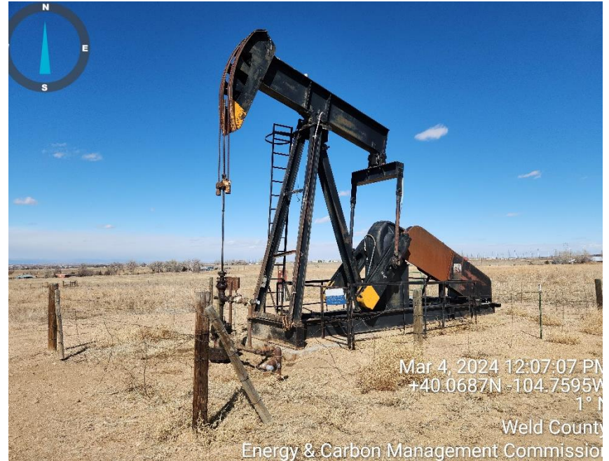
Photo 2 well head and equipment
