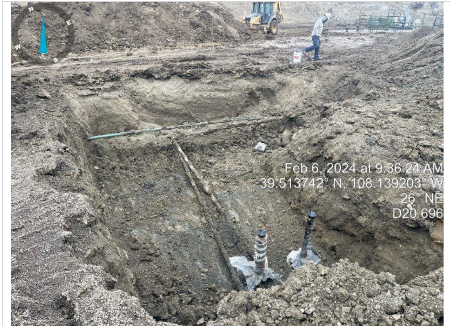
February 6, 2024 - Excavation: Orientation Northeast
