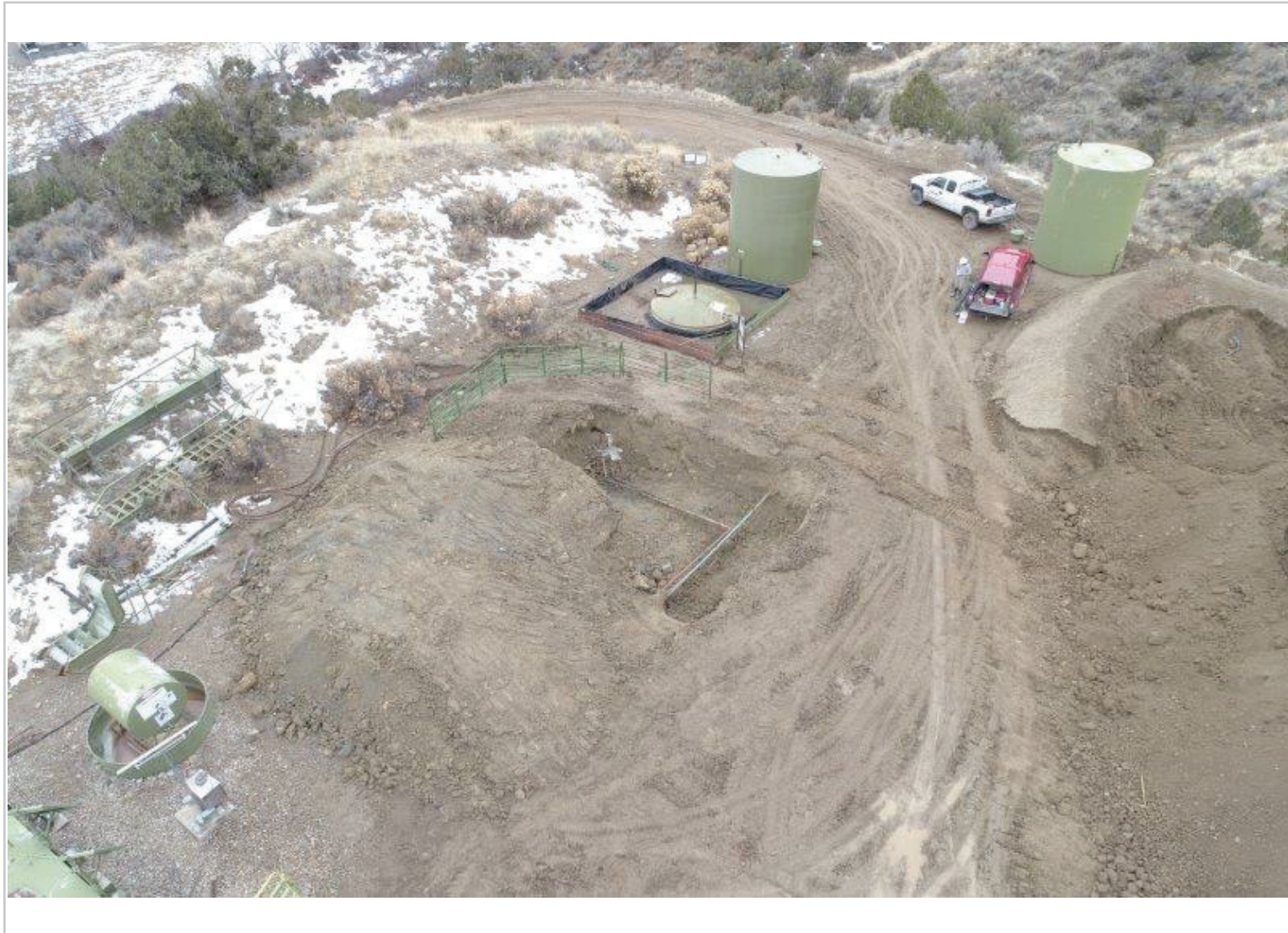
February 6, 2024 - Site Overview: Orientation Southwest
