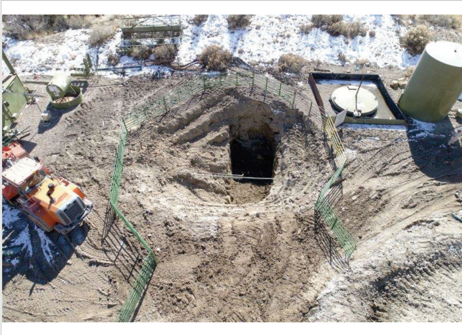
February 13, 2024 - Excavation Overview: Orientation South
