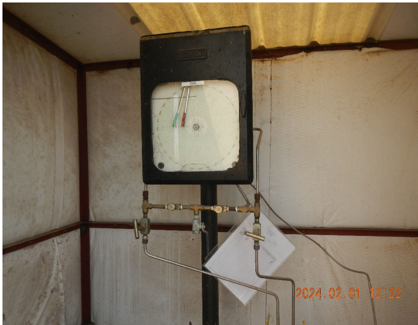
5. Gas meter inside meter shed.
