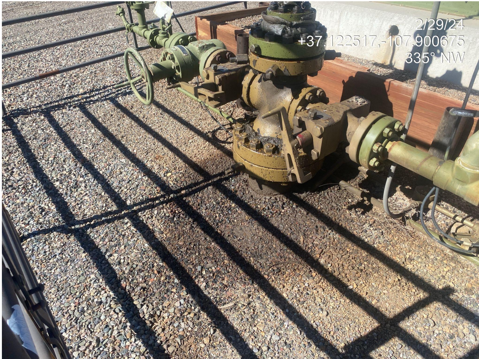
Photo 4. View of impacted surface material observed at well head.
