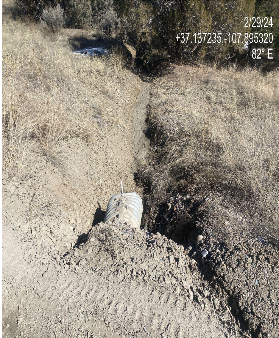
Photo 8. View of culvert that is full of sediment and has not been installed or maintained in accordance with good engineering practices and causing erosion moving east off of the access road.
