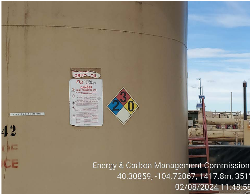
Crude oil tank placards on 2/8/2024
