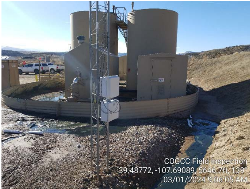
Photo #3 – View of released fluids entering perimeter ditch on north/northwest end of pad, looking South. Note absorbent booms had been installed by Operator prior to inspection.
