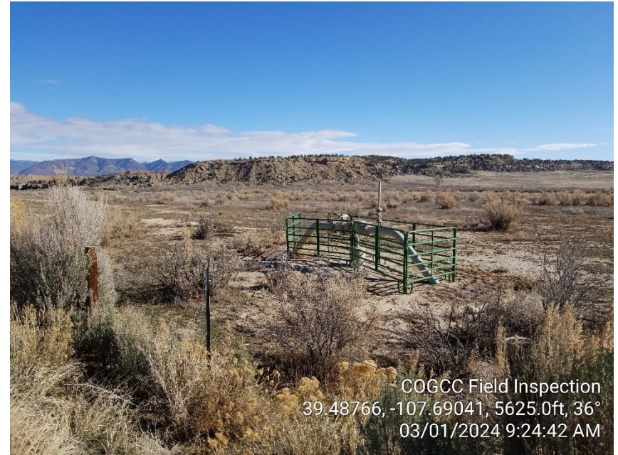
Photo #8 – Pig launcher located approximately 170' Northeast of the observed point of release, across C.R. 315. During inspection, ECMC inspector observed areas parallel to flow path on the opposite side of C.R. 315 with Operator. Unidentified fluids were observed at the pig launcher, but no hydrocarbon stains, sheens, or odors were observed in area.
