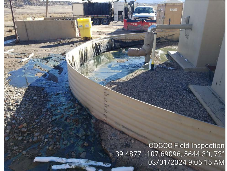
Photo #2 – Fluid release at north end of tank battery, looking east. Note presence of fluids inside of tank battery secondary containment area and just outside of containment to the north/northwest.
