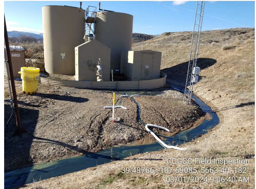
Photo #4 – Released fluids inside of perimeter ditch on north end of facility.
