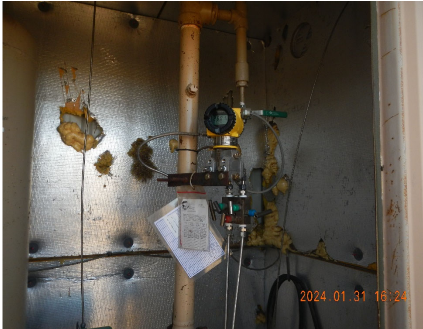
7. Digital gas meter inside remote meter shed.
