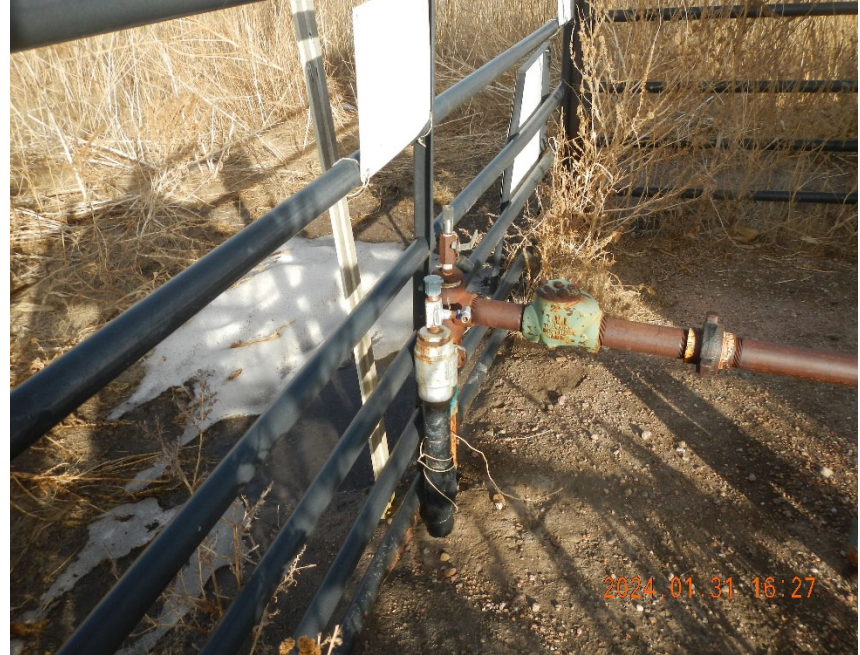
6. Flowline riser and valve located at remote metering location.
