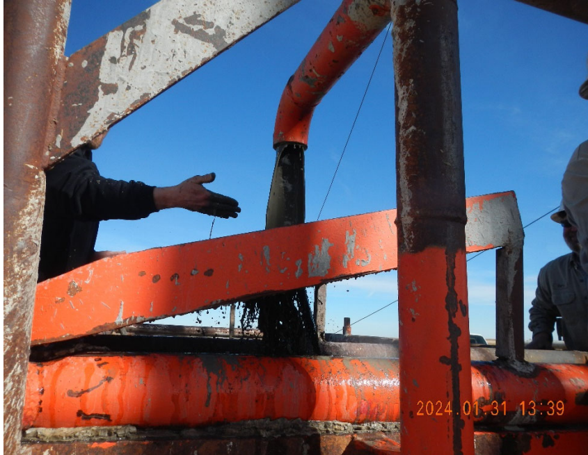
5. Cement returns to surface as cementing annulus space for repair is completed.
