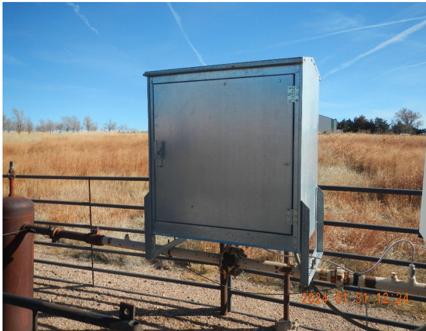
3. Flowline mounted gas meter box.
