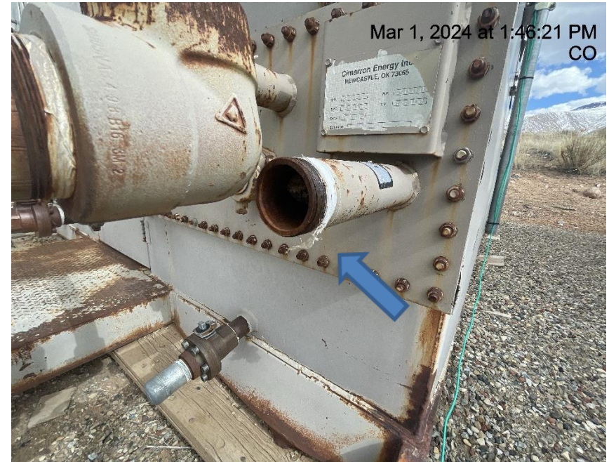
Photo # 8155 Open ended pipe on production separator/wildlife hazard
