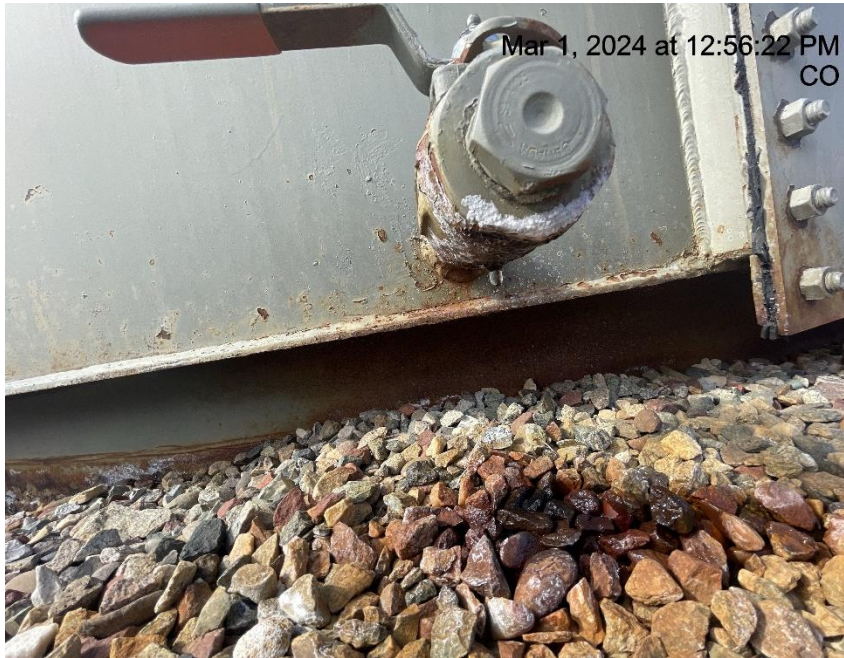
Photo # 8080 Valve on production tank leaking fluid
