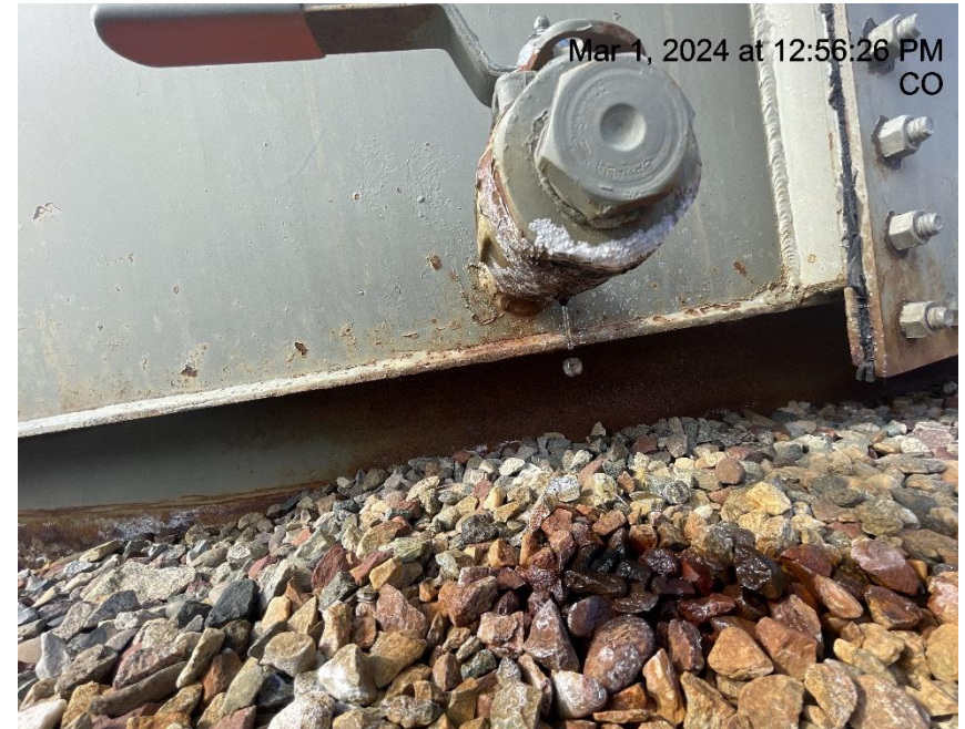
Photo # 8081 Valve on production tank leaking fluid
