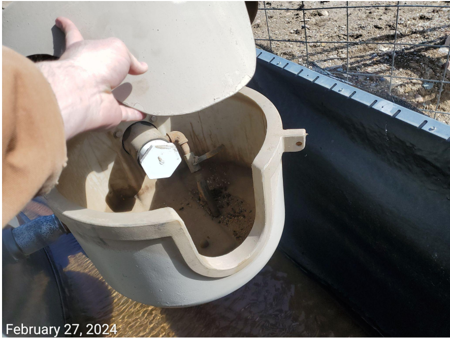
Photo 2: Lines at tank has been capped
