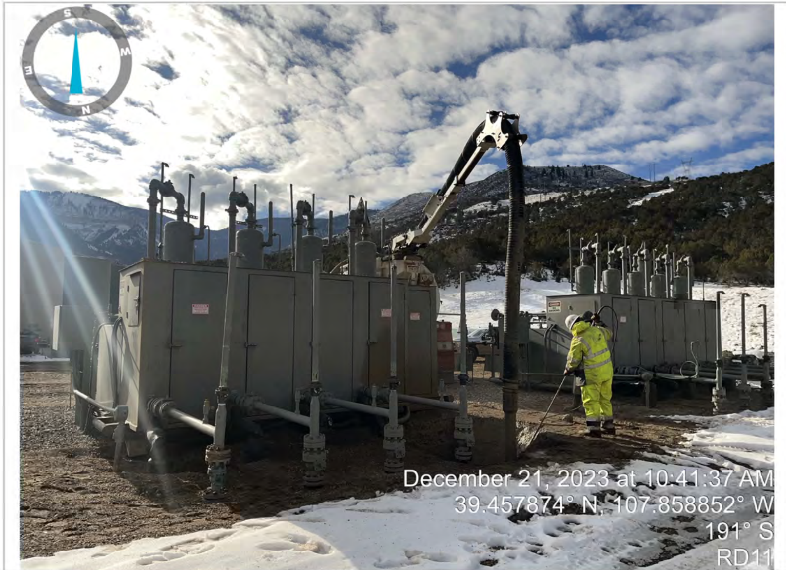
Hydrovac Excavation Point of Release: View South
