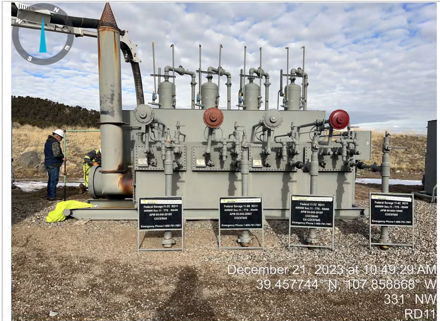
Hydrovac Excavation Point of Release Overview: View Northwest
