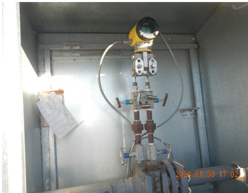
3. Digital gas meter inside meter box.
