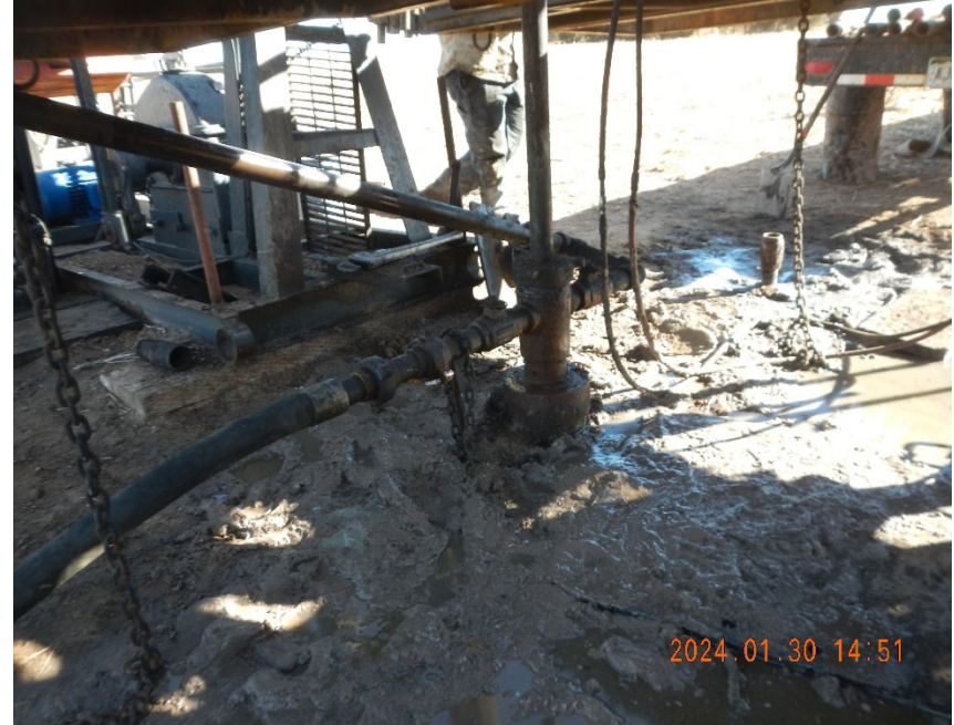
4. View of wellhead set up for pressure testing.
