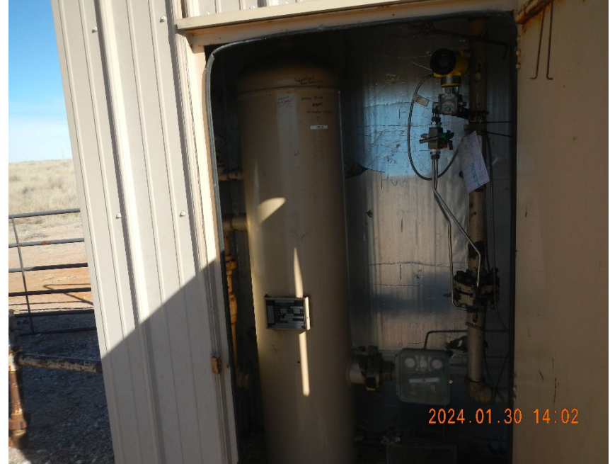
4. View of Separator and gas meter inside shed.
