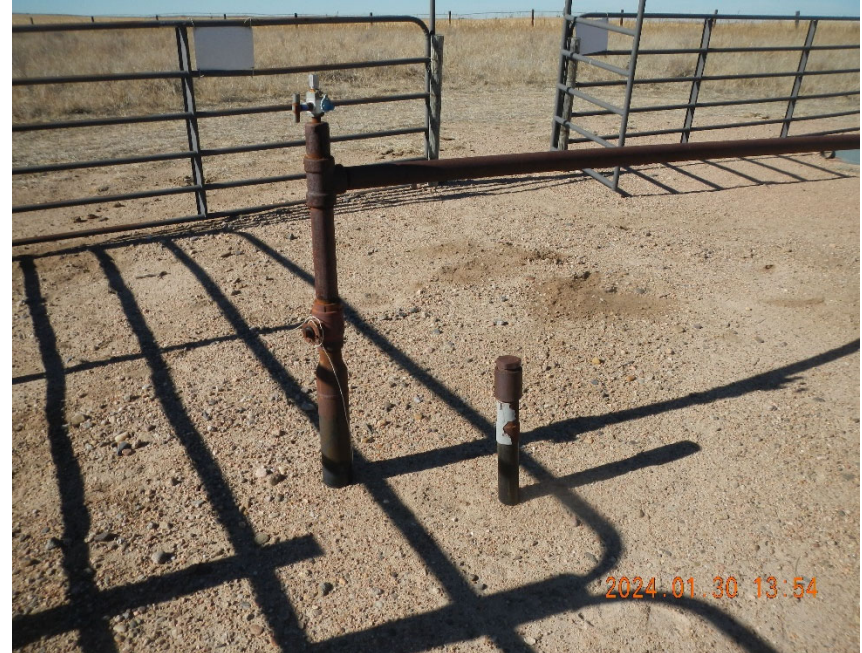
4. Riser with plug at wellhead.
