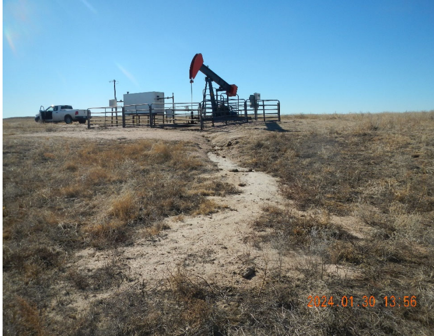
7. View of erosion channel looking back up grade towards well pad.
