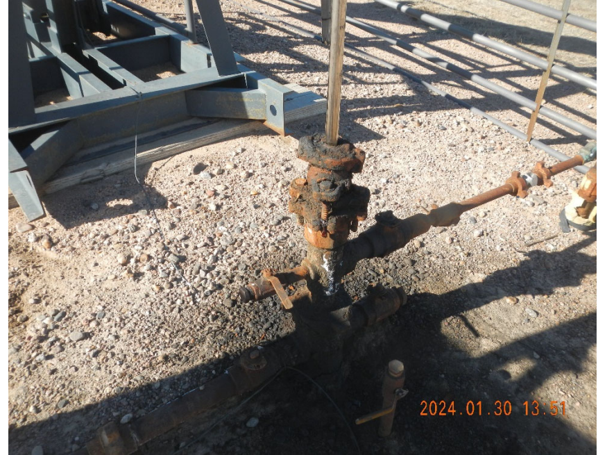
2. View of wellhead. Note staining around wellhead.
