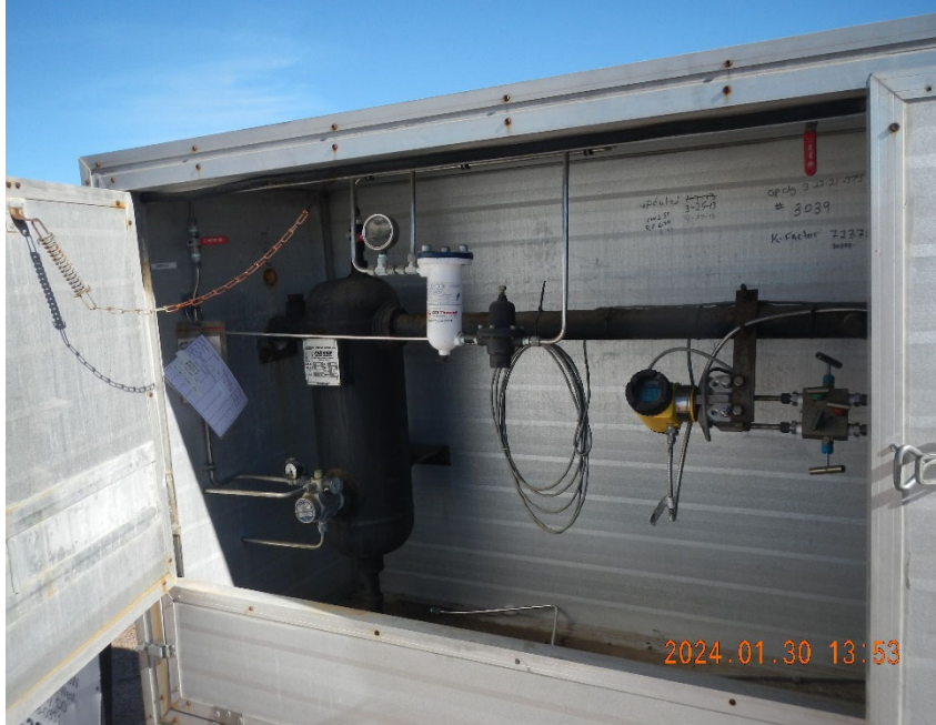
3. Separator and digital gas meter inside meter box.
