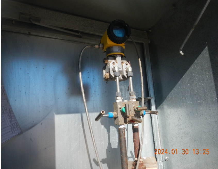
3. Digital meter inside meter box.
