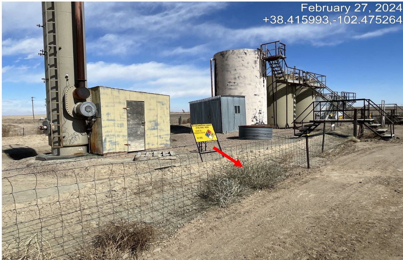
Photo 5. Facing toward the backside of the tank battery. There is blue stained weed debris from recent ground sterilizer applied around the equipment.
