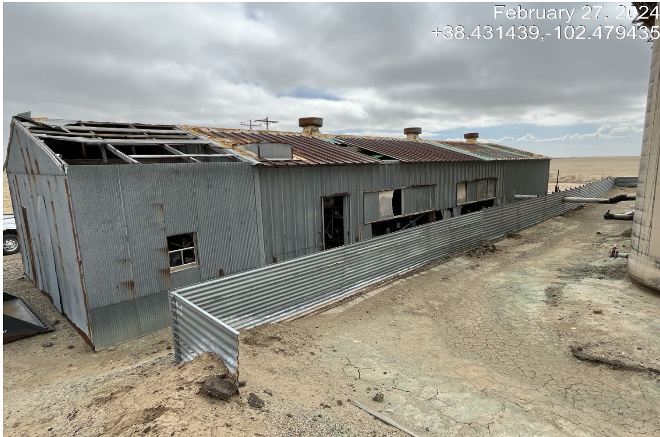
Photo 2. Facing southeast toward the storage shed adjacent to the tank battery. The tin roof has blown off and it appears more of the shed is close to blowing away.
