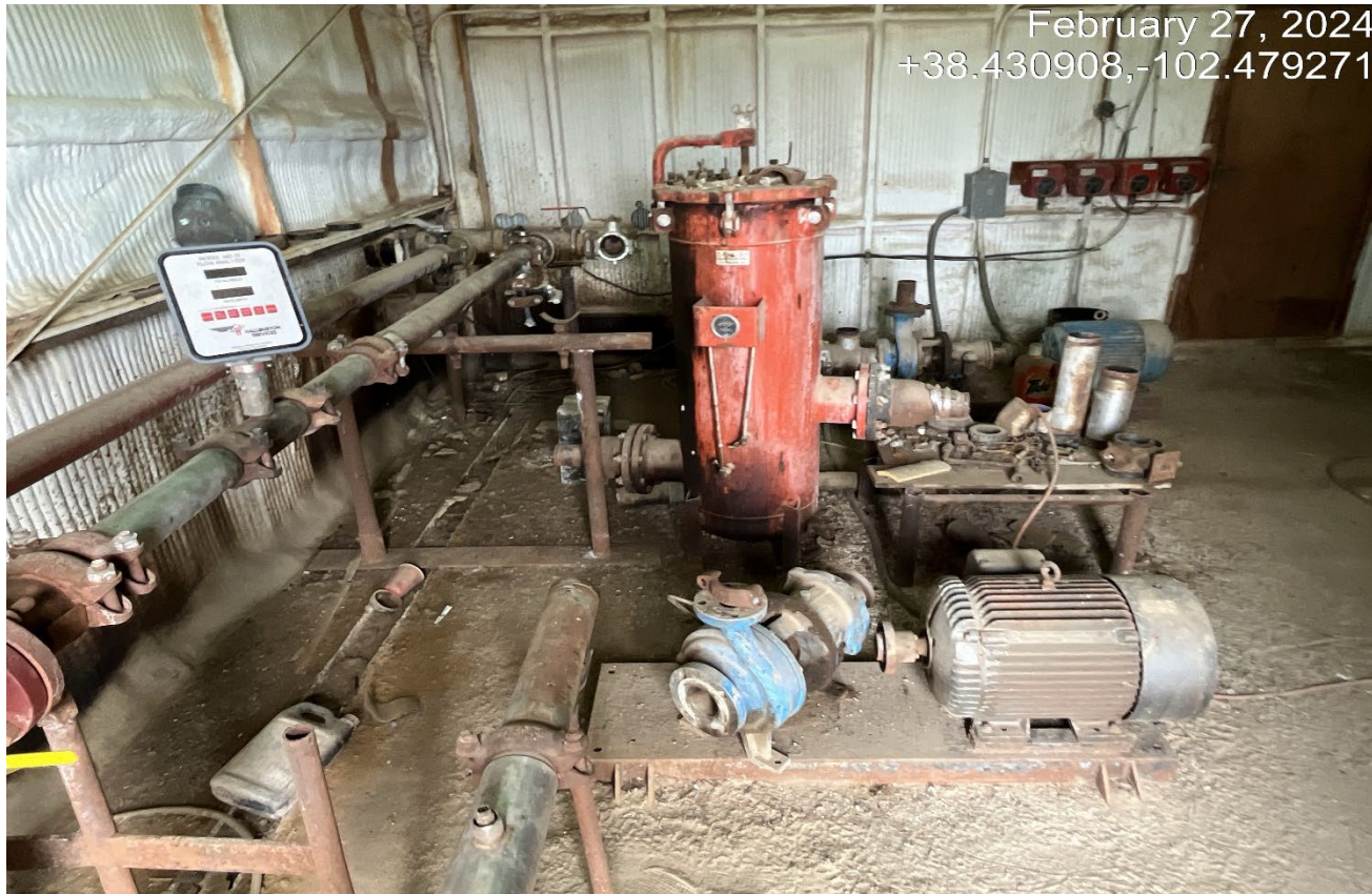
Photo 7. Inside the south end of the building is where flowline meter is located. There appears stained soils around the flowline equipment.
