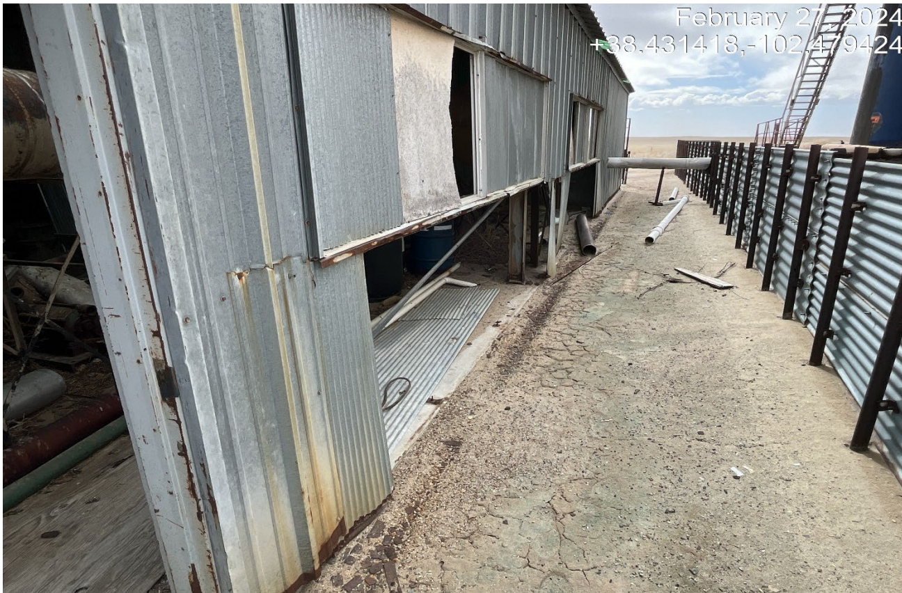
Photo 3. There was pieces of tin rattling and loose along the vack side of the storage shed.
