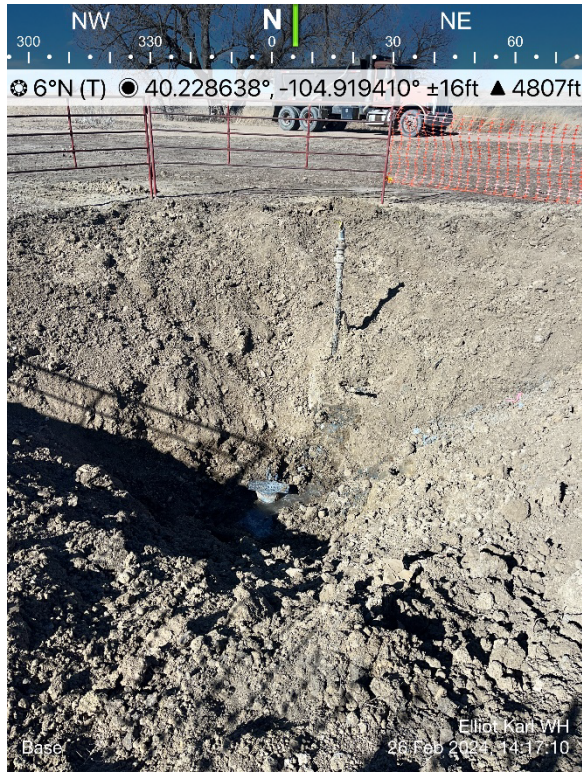
Wellhead Excavation
