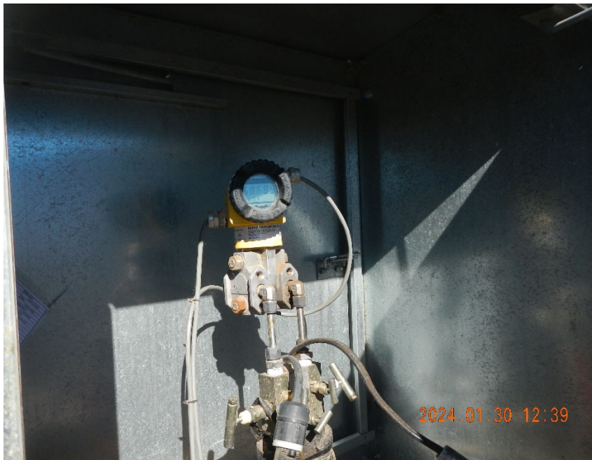
3. Digital gas meter inside meter box.
