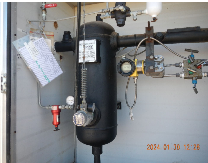
5. Separator and gas meter inside meter box.
