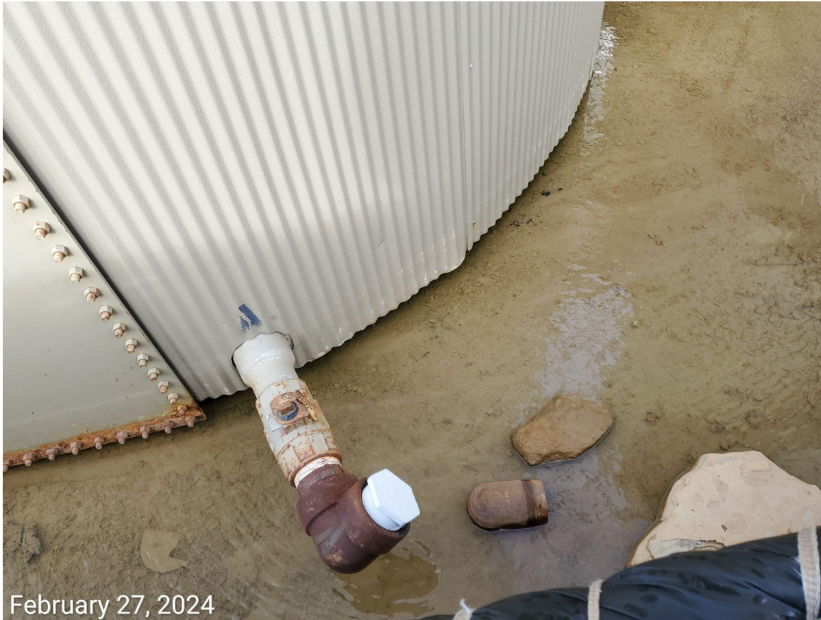
Photo 3: Photo examples showing caps/plugs have been installed at the lines at tanks.
