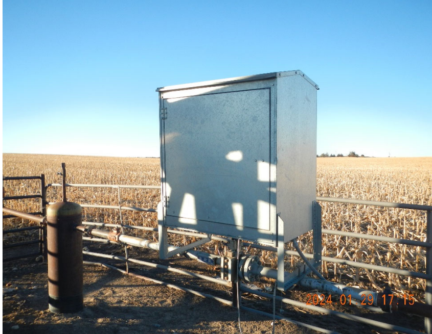
3. Flowline mounted meter run box.
