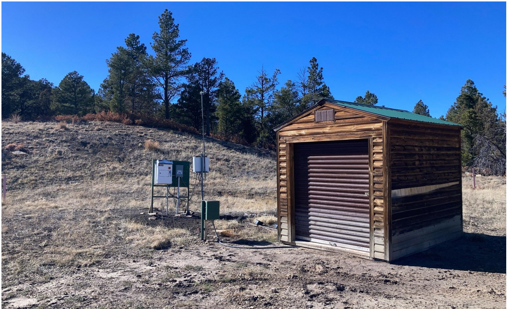
PHOTO 3: WELLHEAD AND EQUIPMENT
